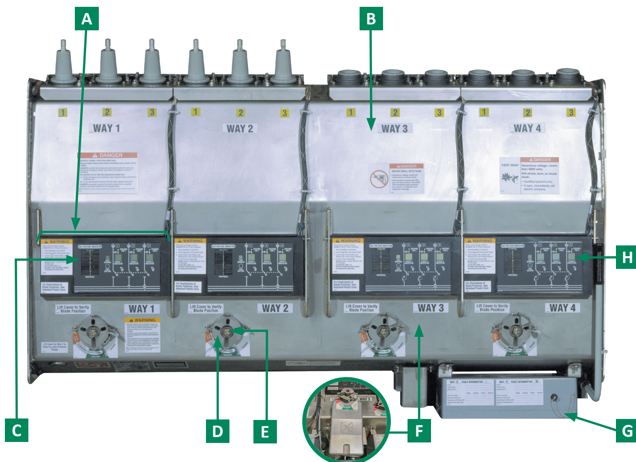
FIGURE 2. Vista and Vista Green Underground Distribution Switchgear
