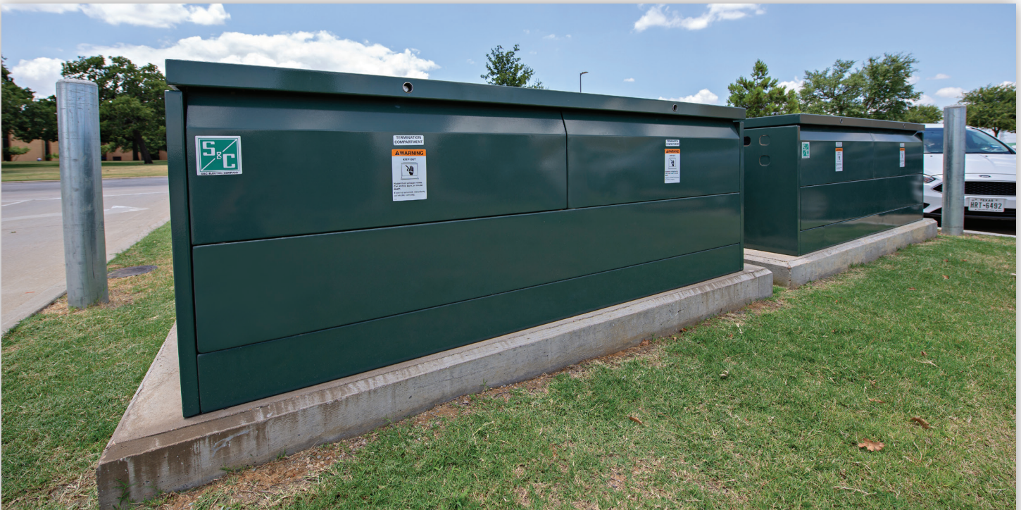
FIGURE 1. Two pad-mount Vista switchgear units.
